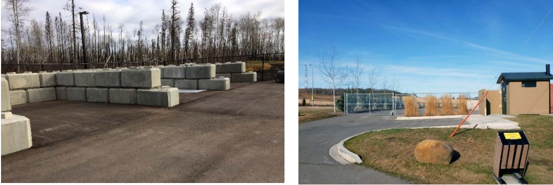
Figure 31. Examples of cemetery operations yards with materials storage bays.
