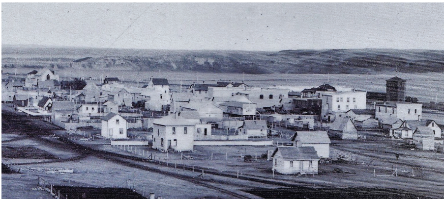
4.1.4(d) Consider the history of diverse roof pitches and styles in Cochrane’s Old Town, seen here from the northwest in 1910, when designing a new building. (Fig. 45: Cochrane Historical and Archival Preservation Society)
