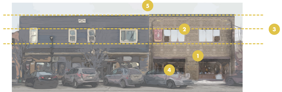
4.1.2(d) The traditional-style building sketch on the right successfully responds to the adjacent Heritage Register building using (1) buff brick cladding; (2) punched windows of a similar scale and orientation; (3) consistent datum lines; (4) retail bays of a similar width; and (5) a flat roof. (Fig. 33: ERA 2020)
