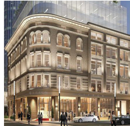
4.1.4(a) A distinct material change is one way to convey the appearance of a smaller-scale building at the streetwall (Fig. 40: Globe and Mail , 2018)
