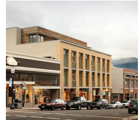
4.1.4(a) An upper-storey stepback is one way to convey the appearance of a smaller-scale building at the streetwall (Fig. 41: HOLST Architects , 2006)
