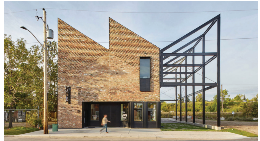
4.2.2(c) Buildings (and site landscapes) can be designed to create subtle interpretations of historic forms and themes, e.g. an interpretation of industrial railway-side building forms. (Fig. 80: Robert Lemermeyer, 2019)
