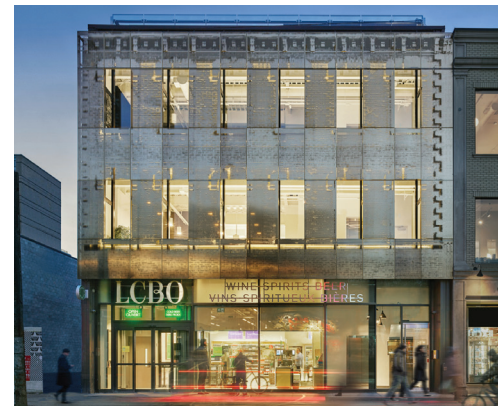
4.1.4(e) An imprinted screen on the upper floors of a contemporary building references the facade of an earlier building on site, since lost (Fig. 46: Quadrangle, 2016)
