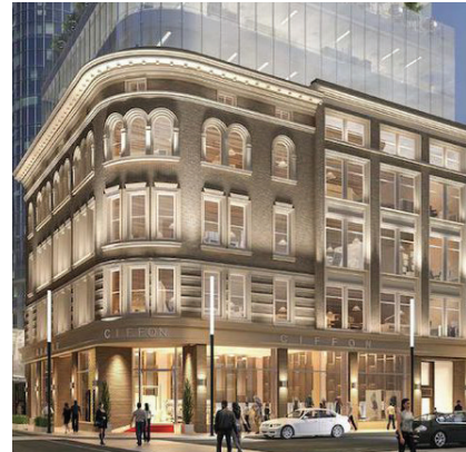
4.1.4(a) A distinct material change is one way to convey the appearance of a smaller-scale building at the streetwall (Fig. 40: Globe and Mail , 2018)
