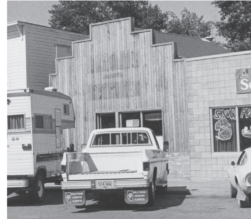
4.1.4(d) A false-front parapet was an historic method of converting a residential building (with a pitched roof) into a commercial storefront. The false front was meant to make the building appear as though it had a flat roof. (Fig. 44: Glenbow Archives, PA-1599-573-107)
