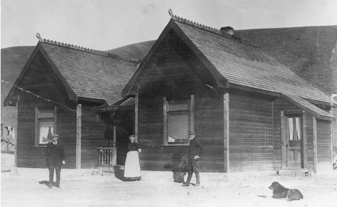
Hospital at Cochrane ,c. 1900-1910. Glenbow Archives NA 854-2
